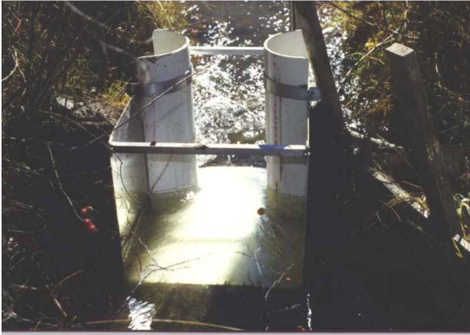
Fig. 3. S-M flume installed in a Northern New Mexico ditch.
