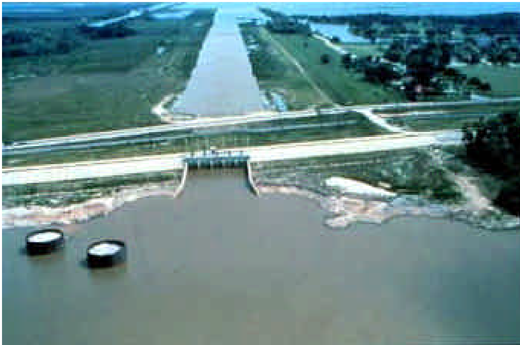
Fig. 2. The Caernarvon diversion structure
